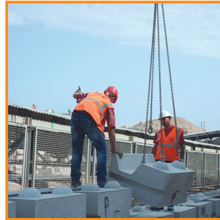
Assembling the Wall
