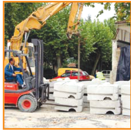
Delivery of the Wall Blocks
