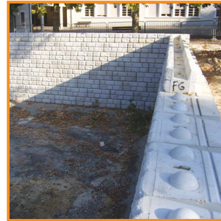
Wall Near Completion
