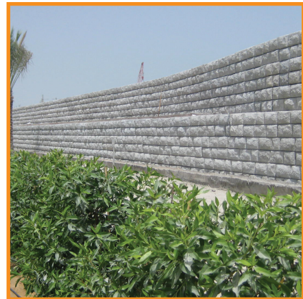
Stepped Retaining Wall
