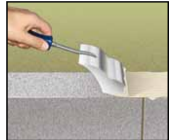
Thin joint mortar being applied with a serrated scoop.
