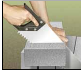
Clean accurate cuts can be achieved using a specific style handsaw.
